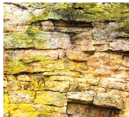
Limestone wall at Swaddywell
