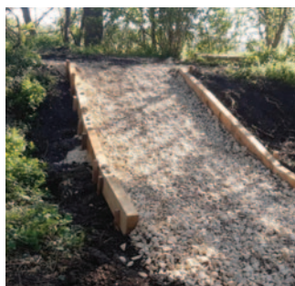
An access ramp
